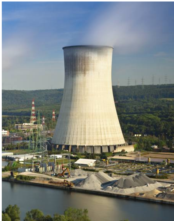
Fig. 11.22. Cooling tower in the form of a hyperboloid.
